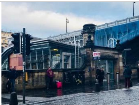
Waverley train station south entrance.
